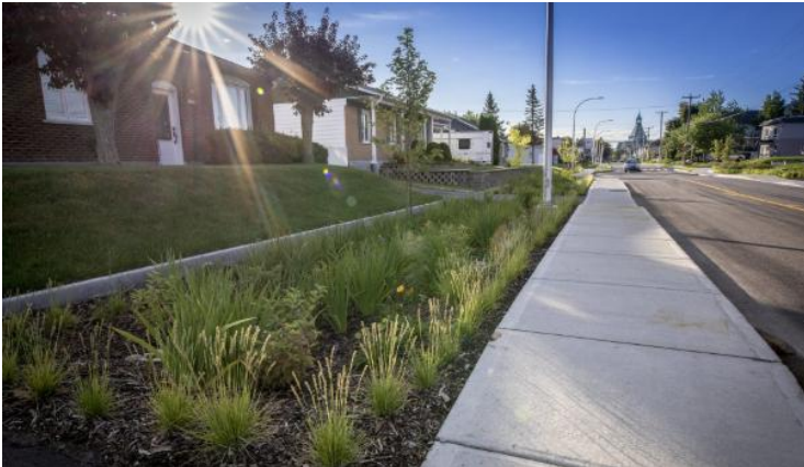
Greening to Improve Stormwater Management
